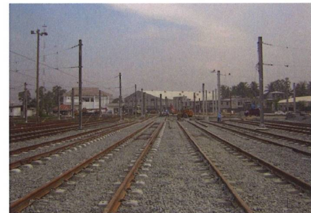
Project: Manila LRT Line1 Location: Manila, Philippines Length: L=2,700m Turn Out 18 nos.
