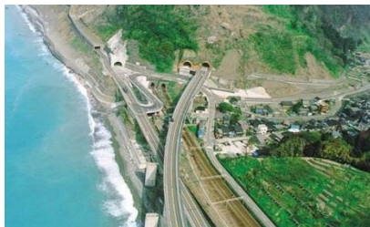
Koshirazu Tunnel (NIIGATA JAPAN)
