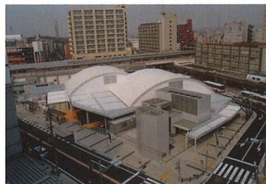
HSST Fujigaoka Station for Tobu Kyuryo Line (Japan)
