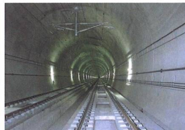
Tohoku High Speed Rail Kindaichi Tunnel (Japan)
