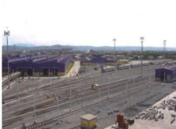
LRT Line2 Depot (Philippines)
