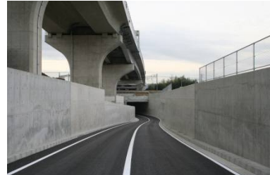
Koshirazu Tunnel (NIIGATA JAPAN)
