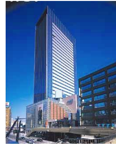
AER Office (MIYAGI JAPAN)
