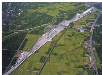
Hokuriku High Speed Rail Depot (Japan)
