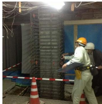
Jacketing of columns
