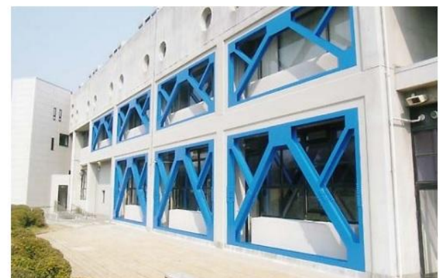
Additional steel braces
